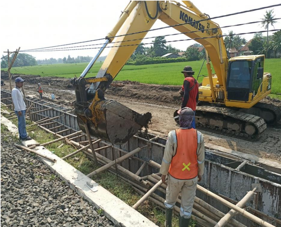
Pek. Pengecoran Body Retaining Wall
