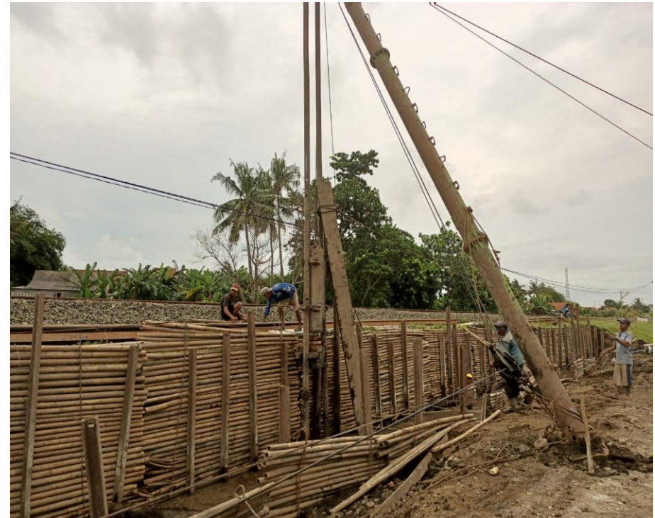
Pek. Pancang MiniPile Retaining Wall
